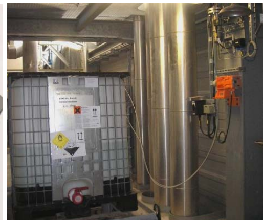
Dosing station for MOL aktiv LM35 treatment
